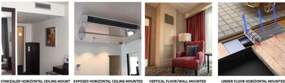
Figure 21. Types of Fan Coil Units
